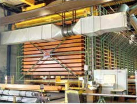
SEW-USECOME, FRANCE Long goods storage system
